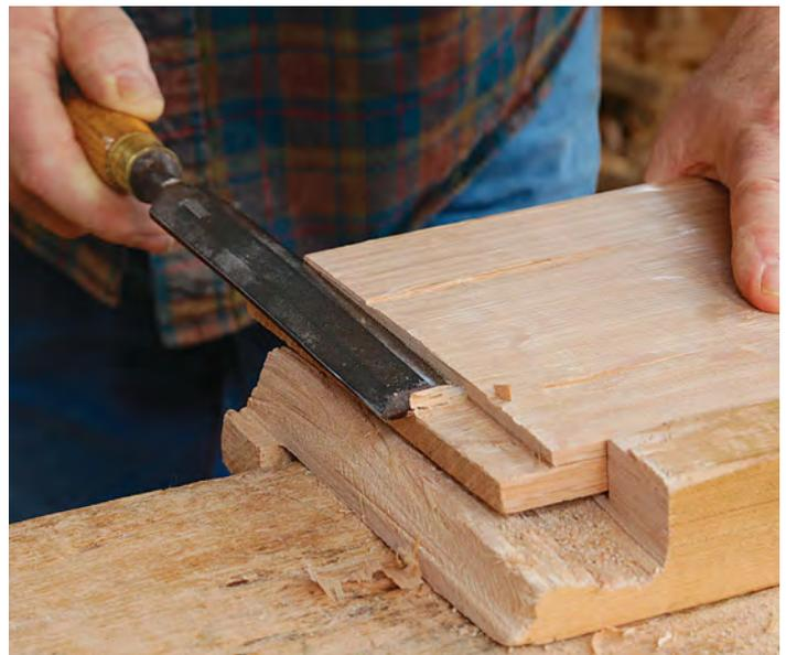
**Pare to the layout line.** Follansbee uses a long paring chisel to flatten the rabbet while bringing it to final depth.
